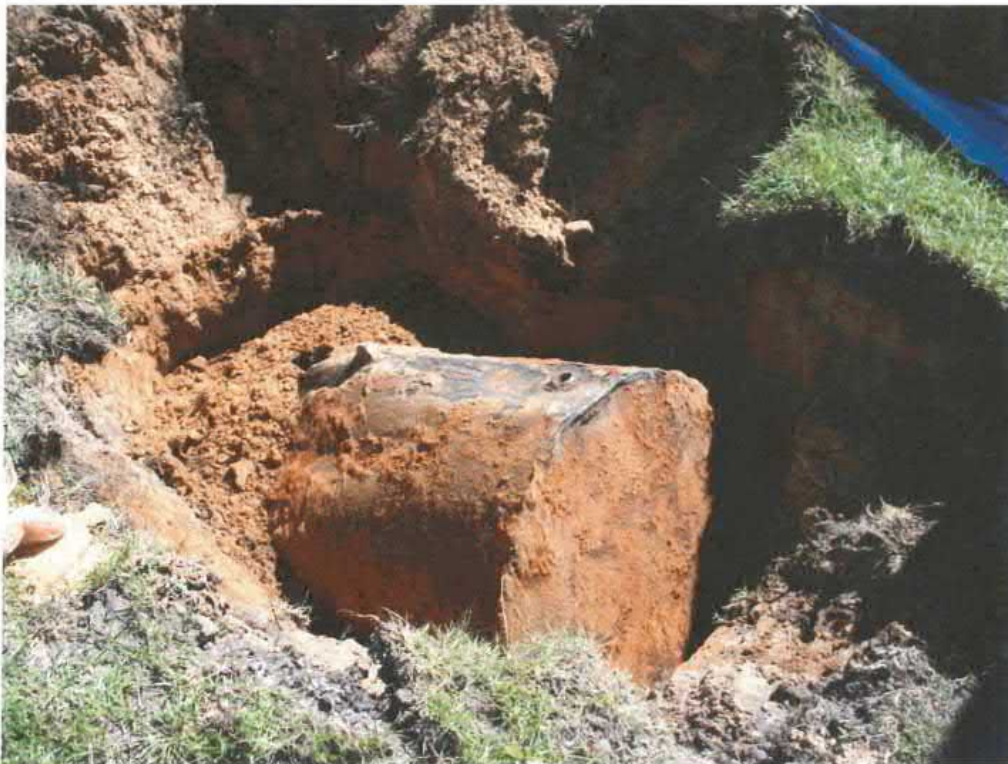
Picture 2: UST 1322Albatross excavation in progress.
